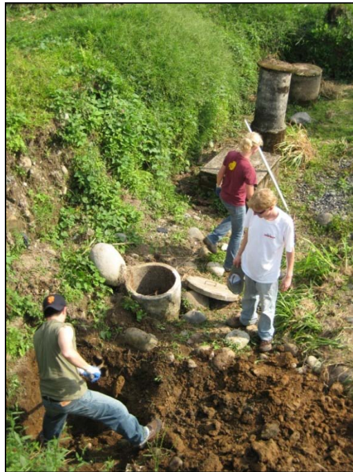
Figure 5: Excavation of Existing Septic Tank
