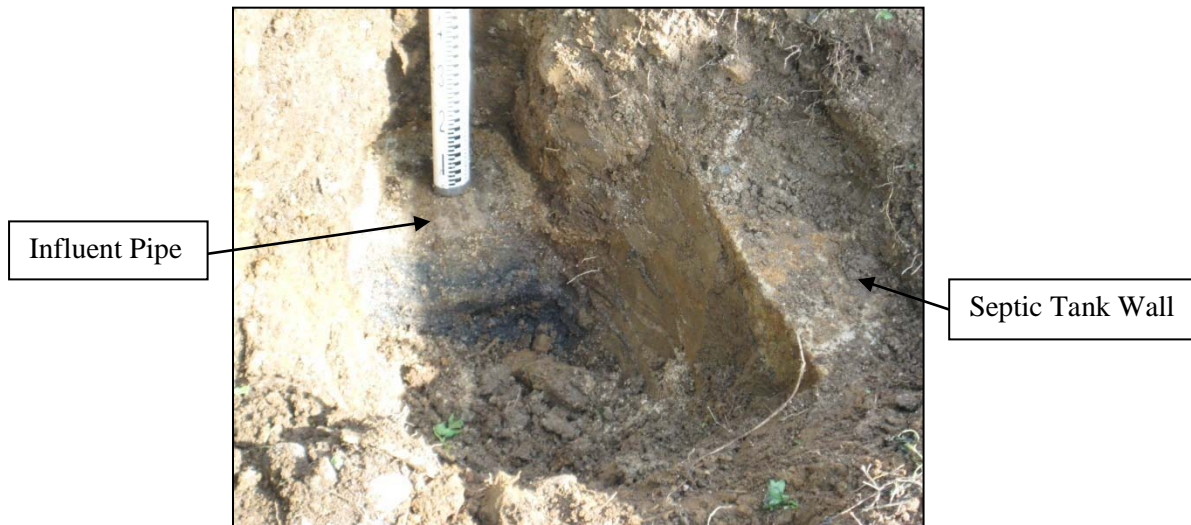
Figure 15: Excavation of Influent Pipe and Current Septic Tank Wall
