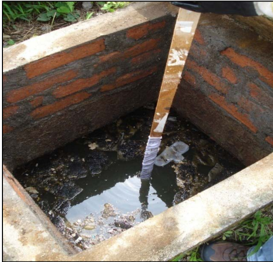
Figure 16: Dipping into center MH
