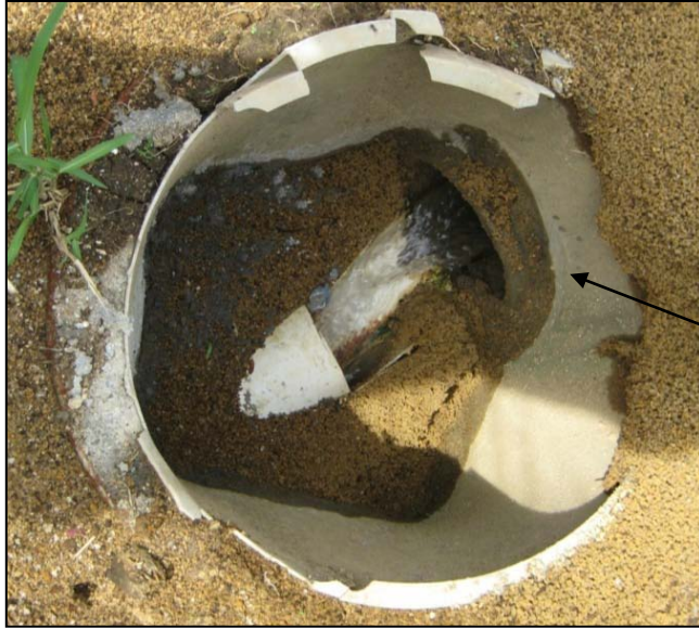
Figure 4: MH5: Broken Pipe and Destroyed Manhole
