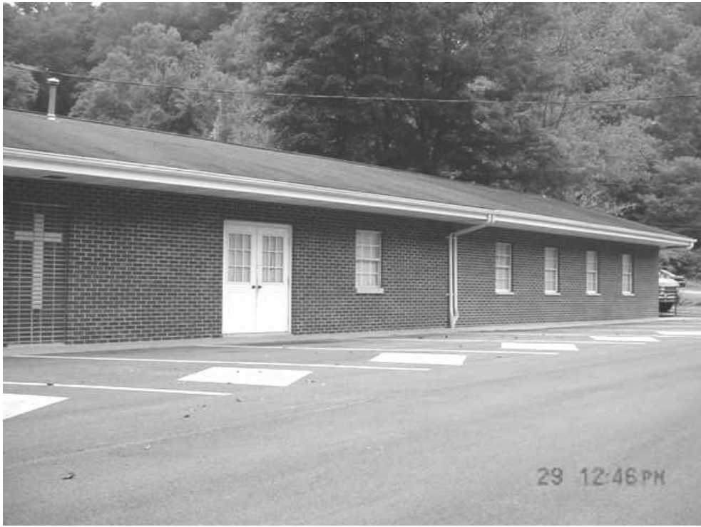
Image 2 - View of the Outside of the Fellowship Hall, Author's Photo
