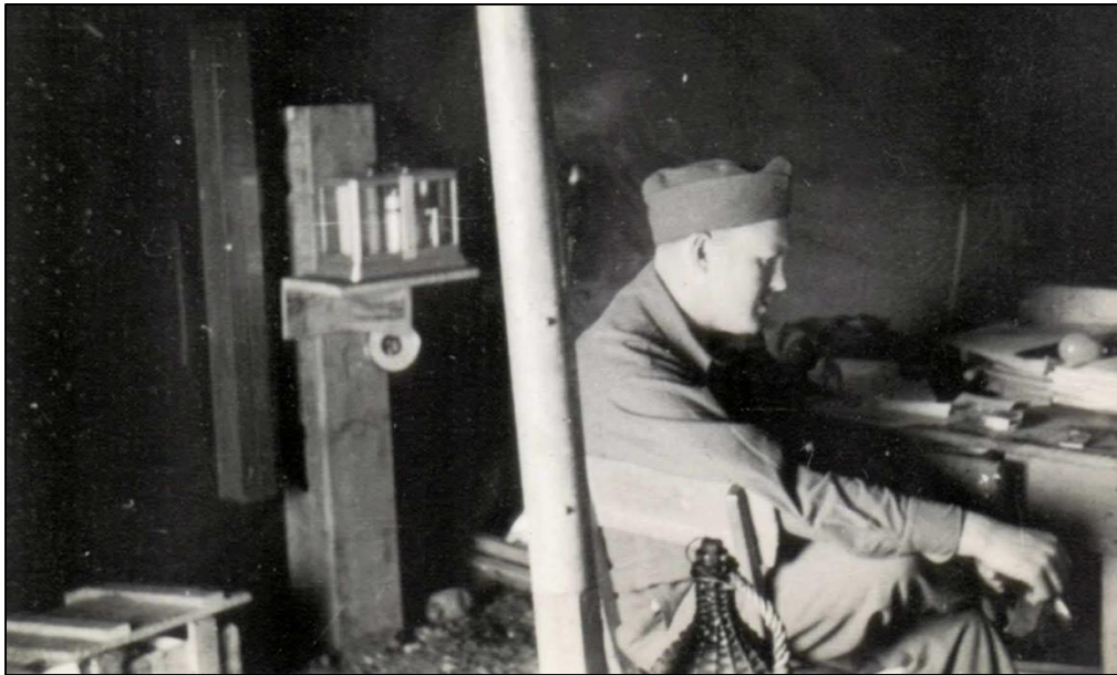
Figure 6. A member of WO Guth's three-man weather team on the island of Vis. Note the barograph in the background, which records pressure readings from an aneroid barometer. Summer 1944. Source: Courtesy, Grey Beret Association.
