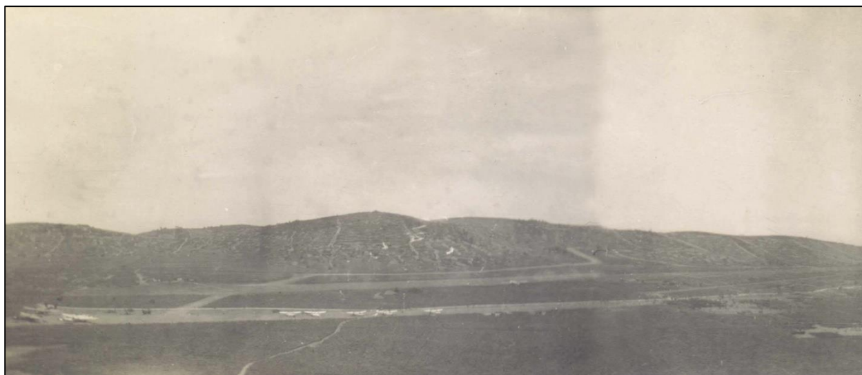
Figure 8. Vis. "American-built airstrip – 4500 ft. Taxi-ways and dispersal areas along hillside. British airstrip enlarged for parking area. Five P-38s in foreground. Three 'Libs' in corner. Tail-less 'Lib' at one edge of main runway. Airport started April 23 [1944], first plane landed April 30 [1944]." Summer 1944.
