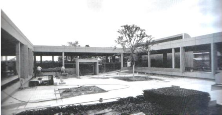
The Gropius addition in course of construction, 1969.
