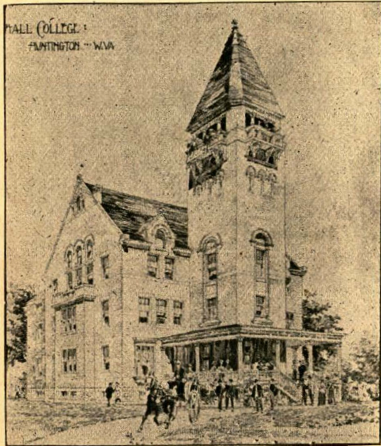
New College Building in Process of Erection.
