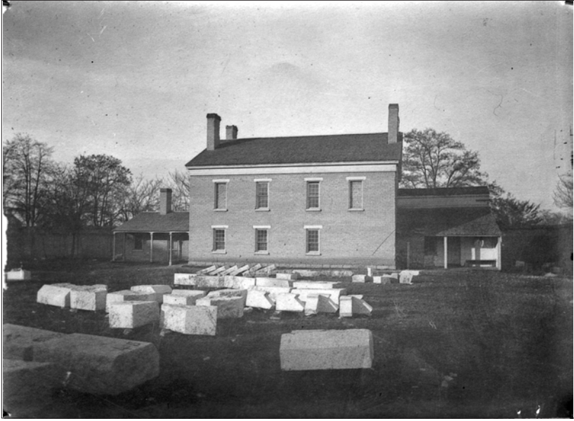
Photo 2. Endowment House, photograph by Charles William Carter, n.d. This photograph has a clear view of the eastern side of the building with its windows and blind windows. The northern extension is to the right. Plainly visible is its frame ridge-line passageway running the length of the extension's top, as well as the dark line on the passageway's extreme right, indicating a slit, or vent, opening into the interior. The door beneath the porch opens into the northern extension's interior. Partially hidden on the left is the one-story southern extension with its interior chimney and porch. Stones for the Salt Lake Temple are in the foreground. Photograph (PH 1300 154) courtesy of the LDS Church Library, Salt Lake City.
