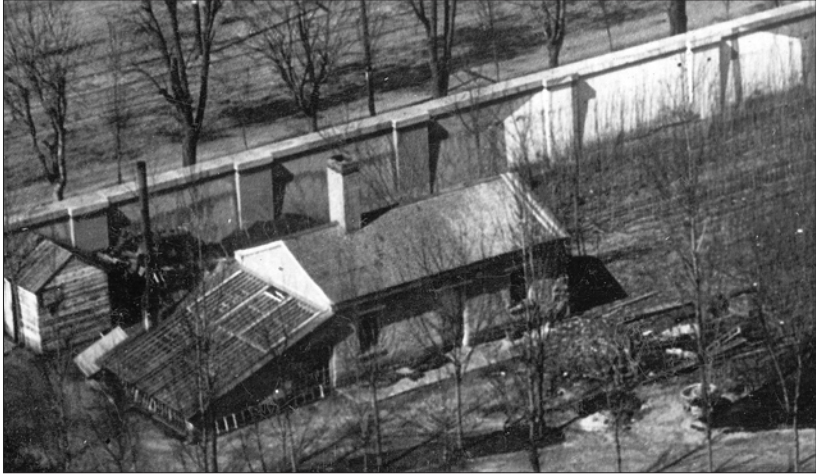
Photo 4. Enlargement of a photograph of the northwestern corner of Temple Square, taken by Charles R. Savage from the roof of the Salt Lake Temple, ca. 1892–93. It shows the southern extension building and its slanted-roof greenhouse, which remained after the demolition of the two-story Endowment House, which had stood where the plowed field is on the right (north). The whitened section on the inside of the west wall of Temple Square (right side of photo) shows where the baptistry had stood. Photograph (MSS P24 Item 496) courtesy of the L. Tom Perry Special Collections, Harold B. Lee Library, Brigham Young University, Provo, Utah.
