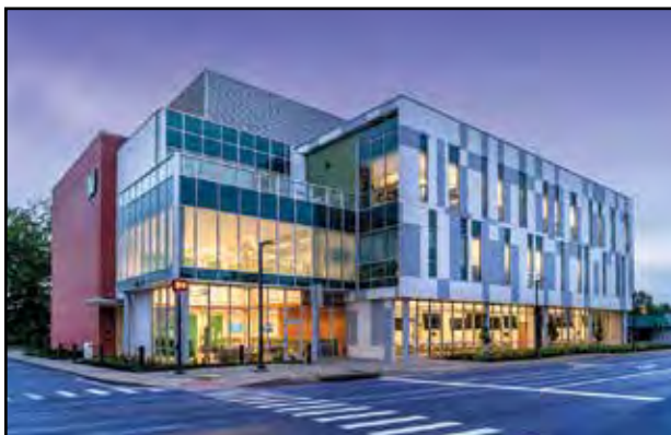
Marshall's School of Pharmacy opened in 2019 as a dedicated, state-of-the-art facility for pharmacy students and faculty.
