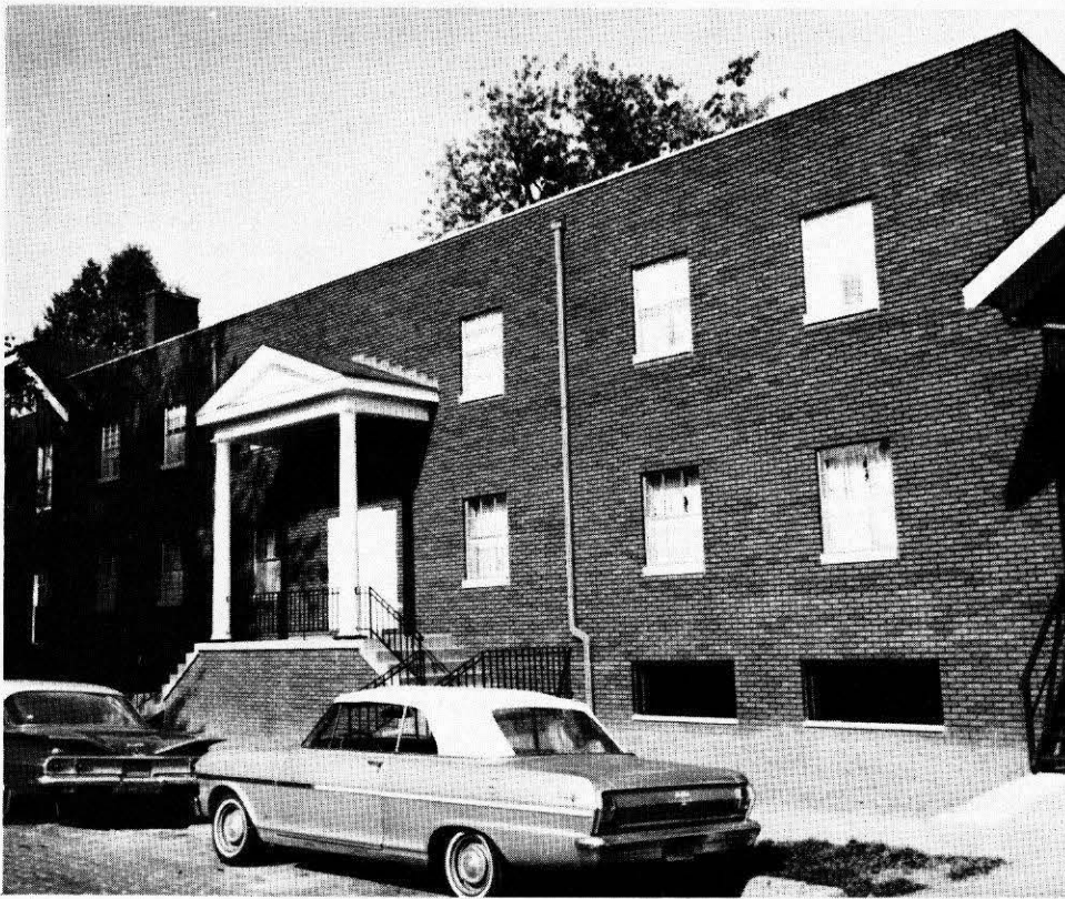
THE NEW ELM STREET entrance to the Alpha Xi Delta sorority house dormitory which was completed this summer and is occupied by some 20 members of the sorority. This new addition cost approximately $50,000.
