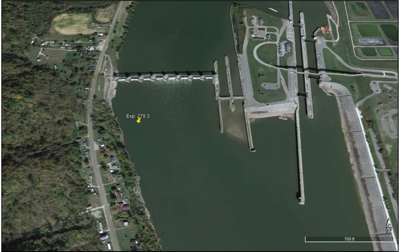
Figure 26. Experimental Site 279.3 and the Robert C. Byrd Lock and Dam Aerial image of site 279.3 showing close proximity to Robert C. Byrd Lock and Dam. Swift water from the tailrace is visible from aerial image.
