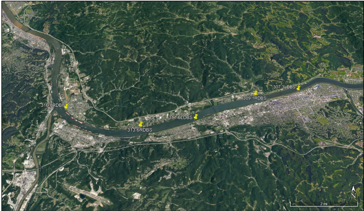
Figure 19. Middle Greenup Pool Sites Aerial image of the middle Greenup Pool sites and surrounding land use.
