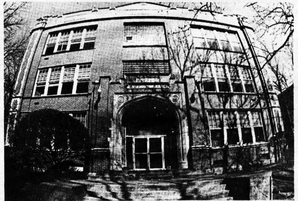
Plans have been submitted to President Robert B. Hayes by Dr. Paul D. Hines, vice president and dean of the Community College, to renovate Northcott Hall into a new central location for the Community College. Photo by Meria Dawson-Broomes
