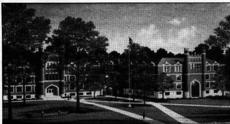
This artist's drawing of the future library shows the view as seen from Hal Greer Boulevard.
