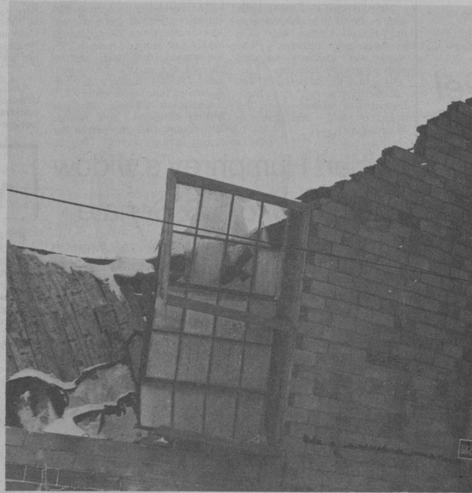
Ruined building still stands after roof collapse
