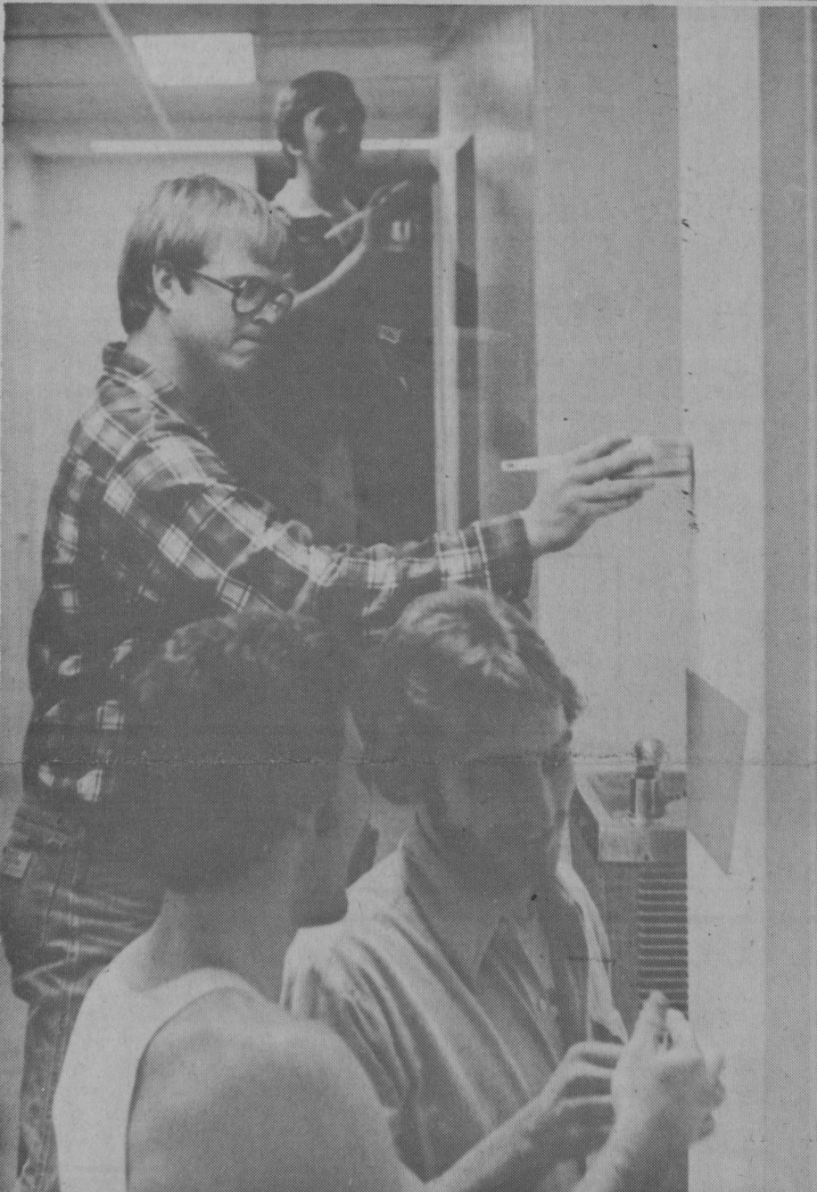
Paintbrushes in hand, these Hodges Hall residents touch up the walls of their "home away from home" during a self-initiated renovation this week. From front, these handy helpers are Joe Sukup, Detroit, Mich.,
