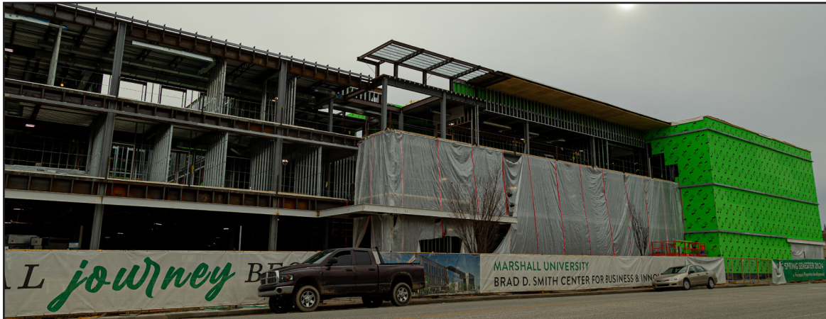
The Brad D. Smith Center for Business & Innovation currently under construction
