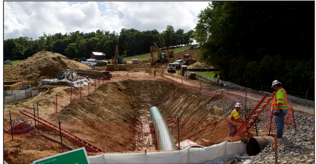
Construction crews are boring beneath U.S. 221 in Roanoke County, Va.
