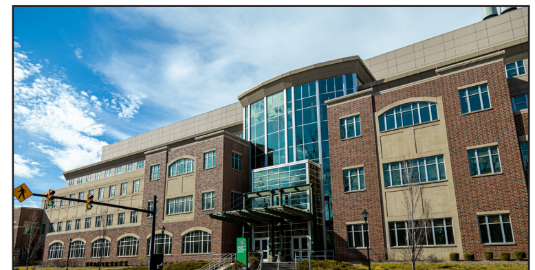
Marshall's Engineering Complex
